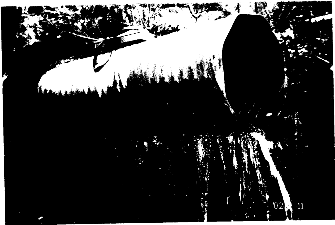
Example of failing culvert on Dement Creek Road
